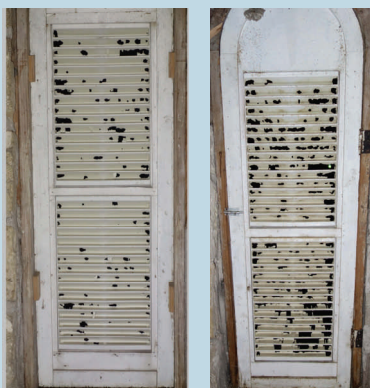
Condition of two ventilating louvers
