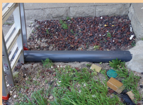
Figure 2. New downspout extension
