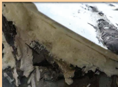
Figure 4. Gap filled with foam.
