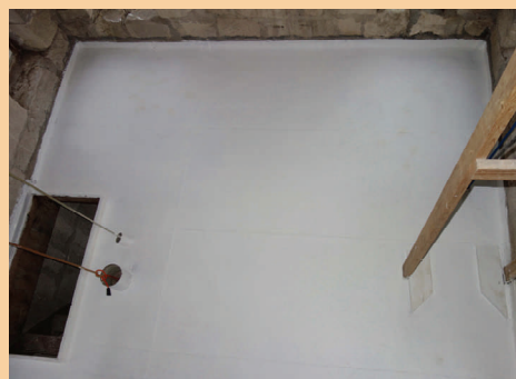
Figure 7. Tin floor cleaned, caulked, & painted.
