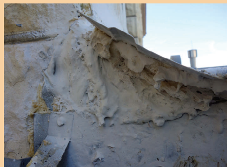
Figure 5. Liquid rubber covering the gap.
