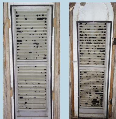
Screens temporarily installed to keep bats out.
