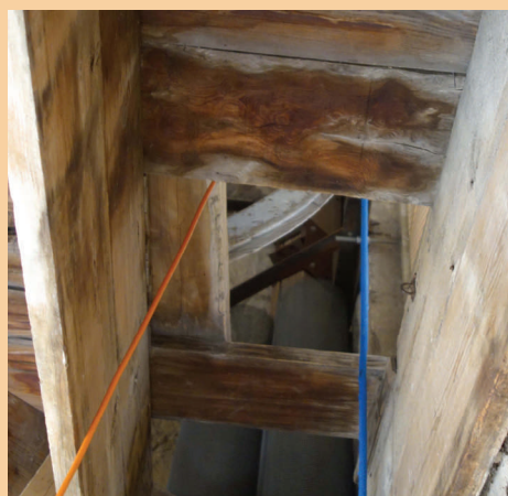
Opening to Bell Tower Floor (21"x 16")
